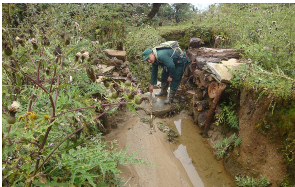
Check dams slowing run-off and retaining soil
